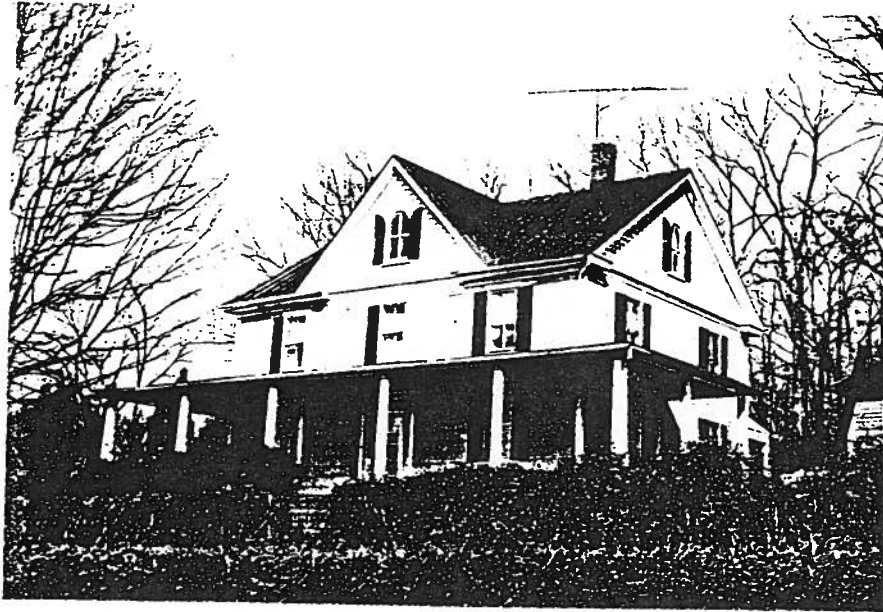
Excellent Two Story turn of the Century Frame Dwelling with predominate Cross Gable. Original sash, shutters, cornice and projecting gable design. Full wrap around one story porch. 53-538 (3497)
