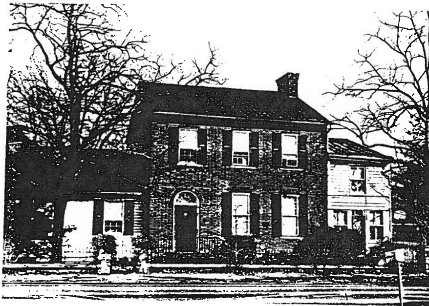
NARROW GATE. Early 1800 two story brick dwelling, with Flemish Bond Brickwork on the front facade. Later frame additions distract somewhat from the original, but the overall quality is good.
