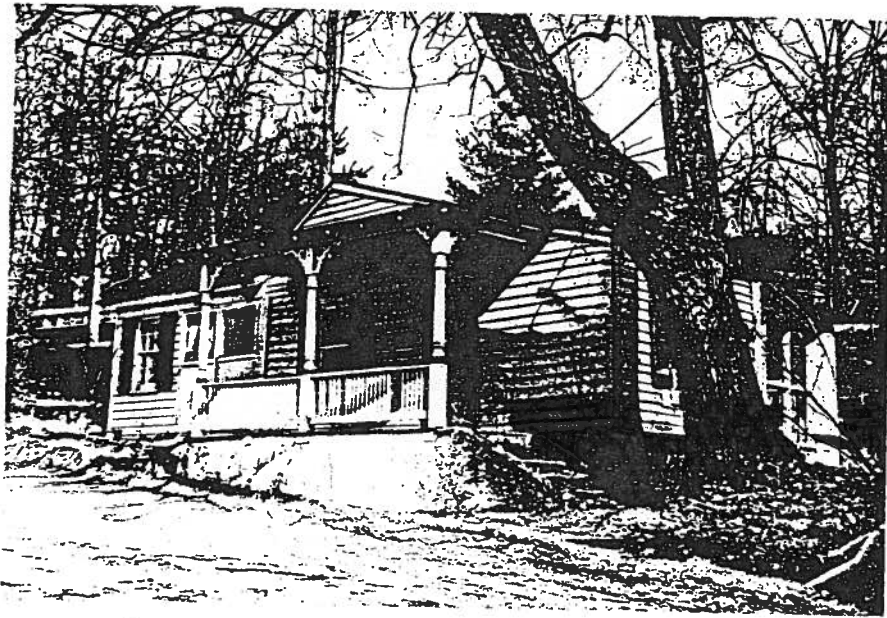
One story frame Dwelling, with pleasing entrance stoop with turned posts and scroll brackets. Original Toll House of the Aldie- Snickersville Turnpike Company, modified into a residence. 53-535
