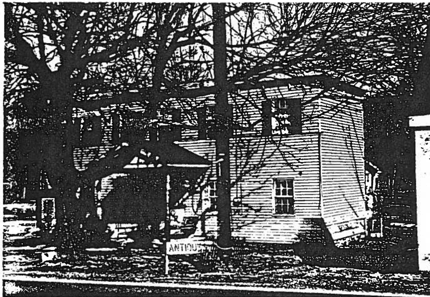
Mid 1800's two story frame Greek Revival style dwelling. May be earlier and modified to this style in the mid 1800's. Good eve Brackets, pleasant entrance porch with turned posts, original sash and shutters. 53-523 (3496)
