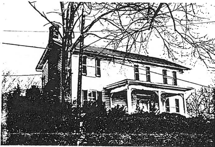
Turn of the Century Two story Frame Dwelling. Original sash and shutters. Good one story entrance porch with sawn brackets. 53-533 (3497)
