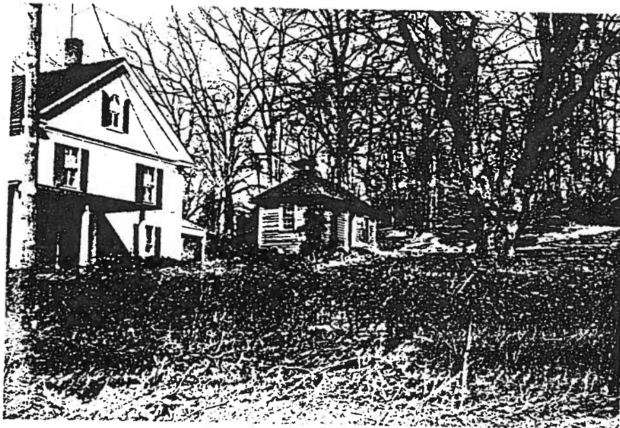
Interesting one story Frame outbuilding. Should be preserved for a suitable use and to retain visual interest. 53-538 (3497)
