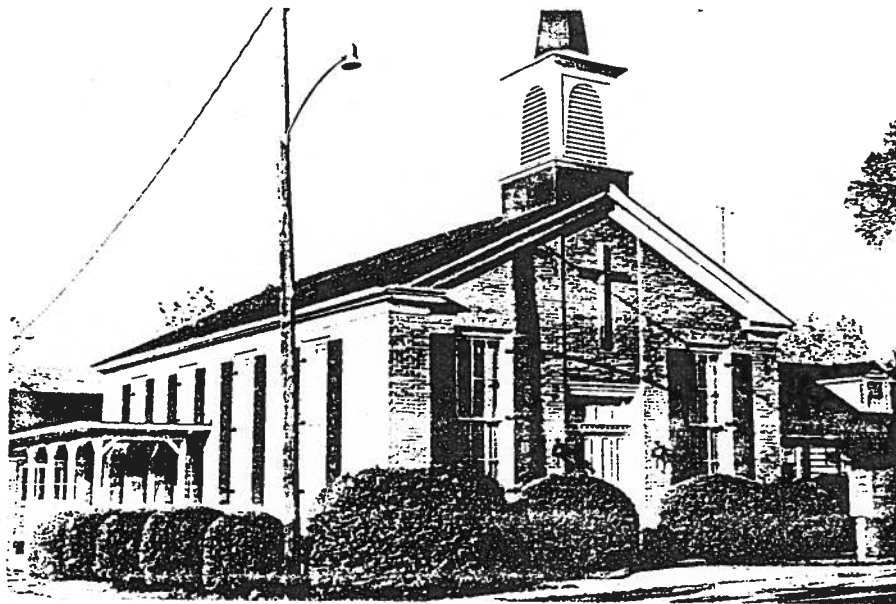
Methodist Church. Built in 1882. Brick veneer was done in 1970 and distracts somewhat from the original quality. Pleasant rural Church structure and worthy of preservation. 53-546 (3503)
