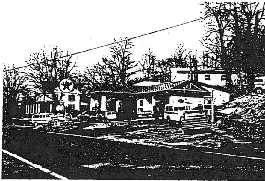
ALDIE GARAGE. Excellent surviving example of a once typical early 1900's Garage and rural store structure. Projecting covered service area should be preserved, if possible. 53-536 (3497)
