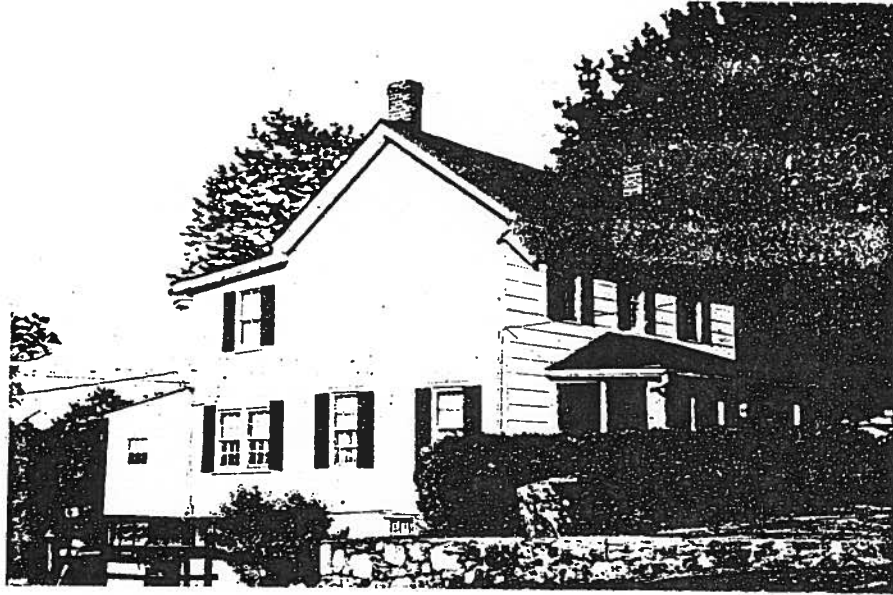
Turn of the Century Two Story Frame Dwelling. Original sash and shutters. Pleasant entrance Stoop. Good state of preservation although shingleing distracts somewhat from the quality. 53-555 (3507)
