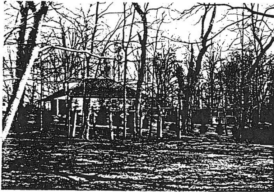
20th Century Stone Tennant house at Berkeley House. One story with hipped roof. Good scale and pleasant design for the area. 53-532 (3496)
