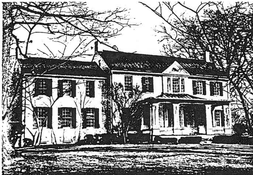
BERKELEY HOUSE. Early 1800's two story Brick dwelling in excellent state of preservation. Pleasantly scaled Pavilion and one story entrance porch with elaborate door unit. 53-532 (3496)
