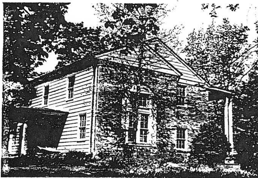
The Weaving House at "ALDIE" Manor. Rear Catslide Roof now modified to a full two story. Now a private dwelling. 53-115 (2617)
